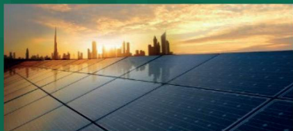
CENTRALE PHOTOVOLTAÏQUE SHEIKH MOHAMED BIN ZAYED DE BLITTA
